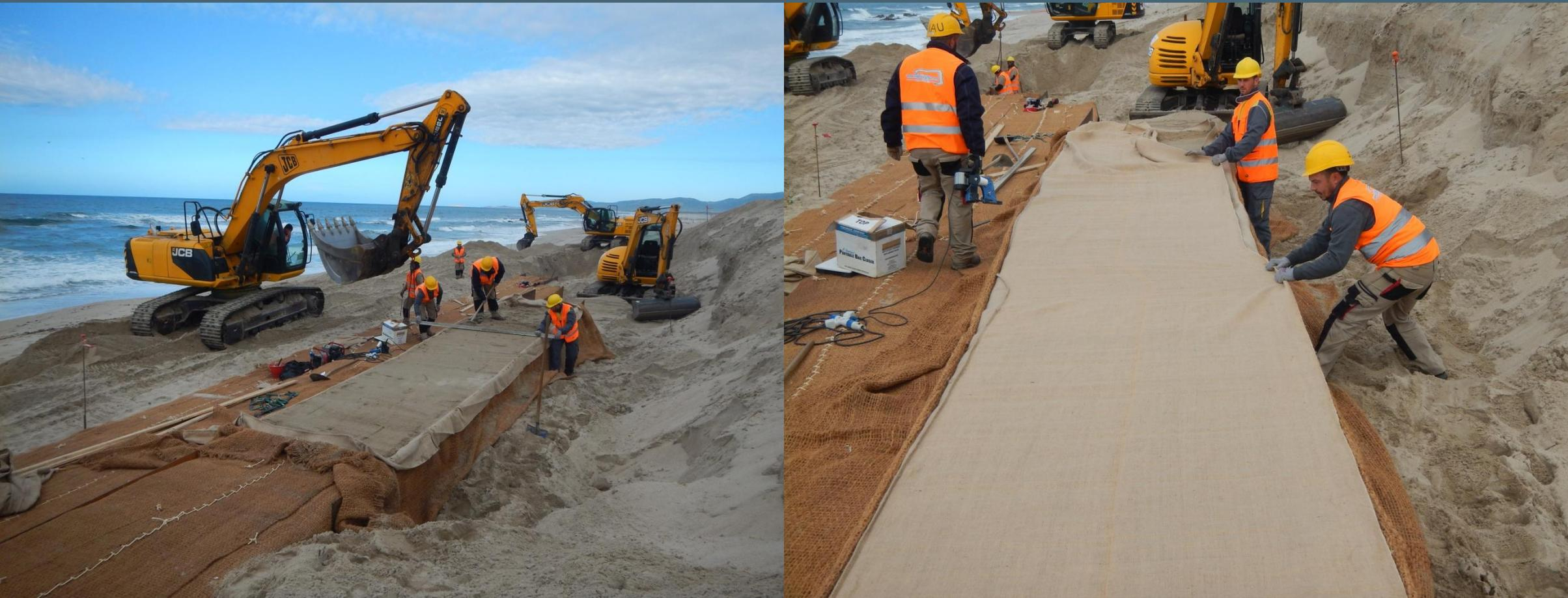
*We were thus able to reconstruct the dune body, set on biodegradable geo-containers, in jute and coconut fiber, filled with local sand, in order to stabilize the dune system temporarily.*
